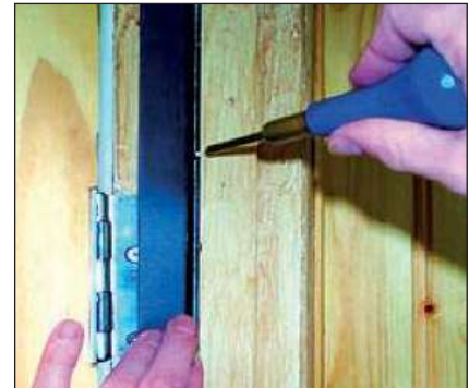
Step 3: Panel pins finish
