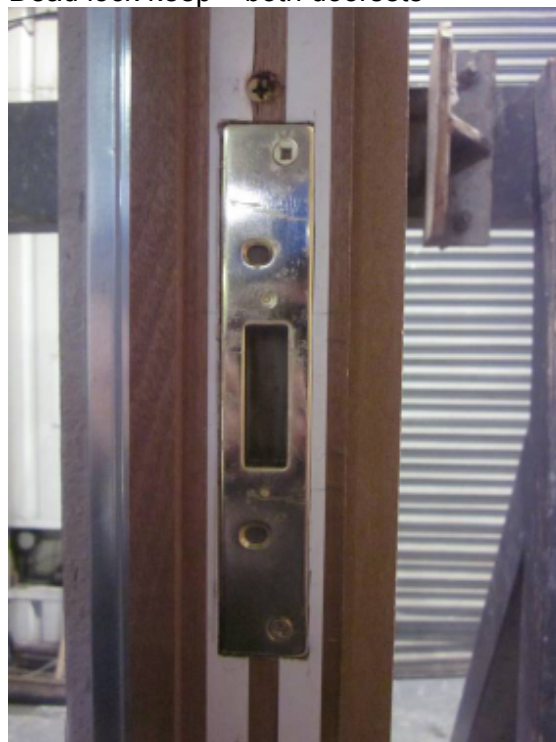
Dead lock keep – both doorsets
