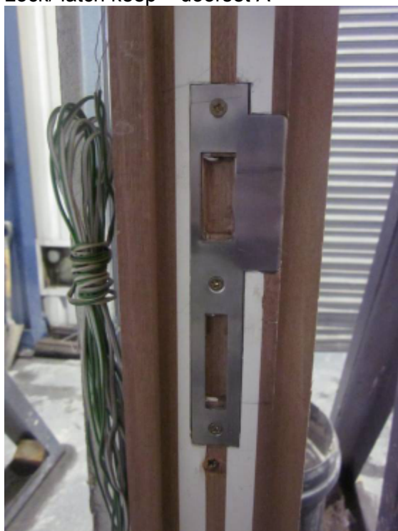
Lock/ latch keep – doorset A
