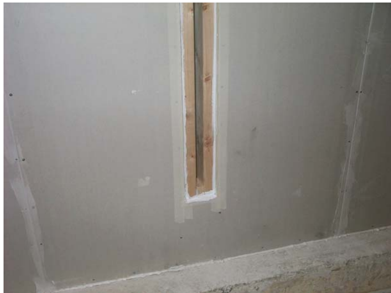
Figure 5 Sealed slot, source room side
