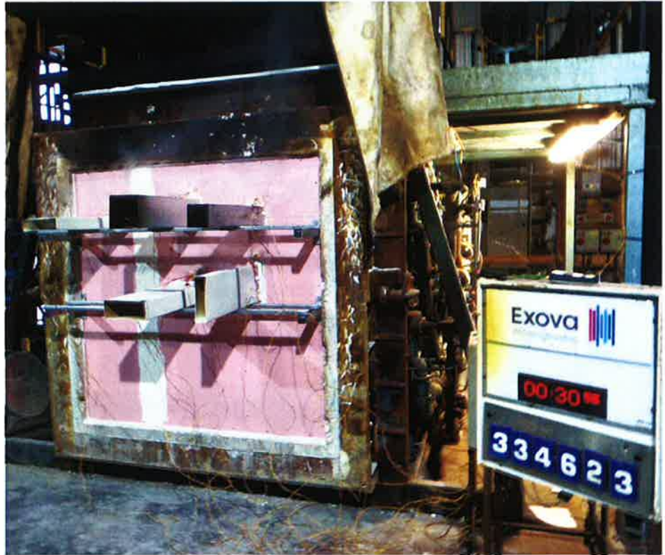
The unexposed face of the test construction after 30 minutes of testing
