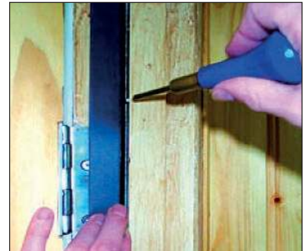
Step 3: Panel pins finish
